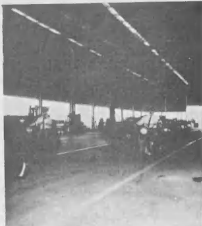
MOTORCADE ENTERS Mechanical shops.
